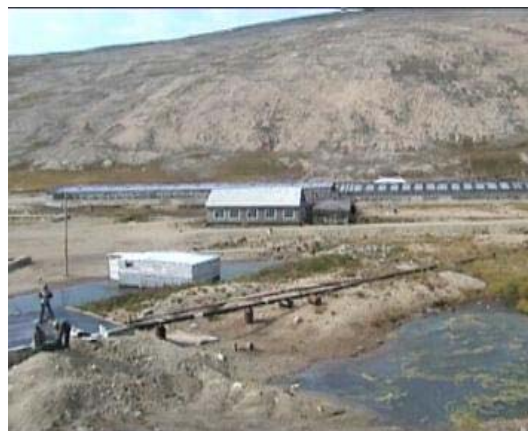
Figure 14: Kukun' (Lorino) Spr. Thermal pipeline on the foreground, greenhouses on the background.
